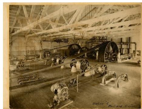
In 1904 **Station C** contained a 800-kW, 550-V railway service generator, rope-driven by a 1,600-horsepower engine; a 750-kW, 10,000-V, 33-cycle generator, rope-driven by a 1,000-horsepower cross-compound condensing engine; and two marine-type, compound steam engines direct connected to a 400-kW and a 200-kW, 550-V railway generator.
